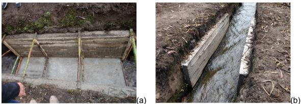
Figure 3: (a) Canal section 24 h after casting, (b) Five months after.
